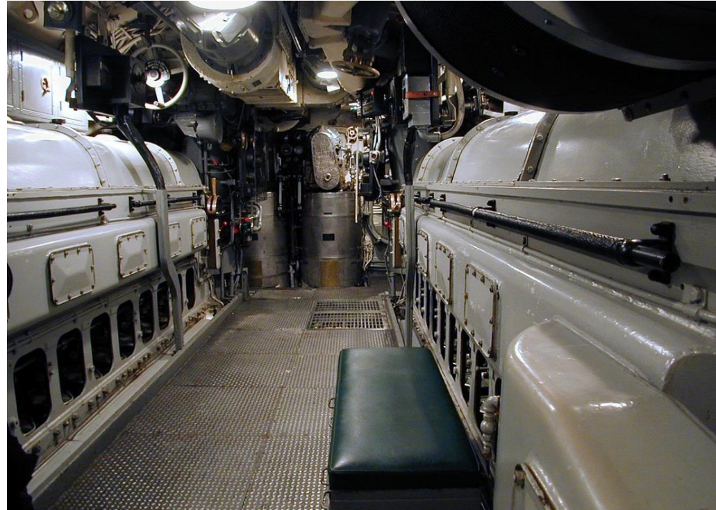
Fairbanks Morse 38 8-1/8 diesel engine on the USS Pampanito submarine
